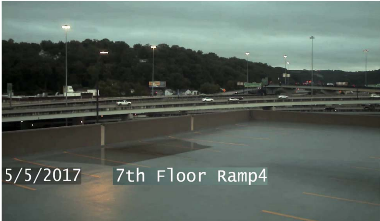
Figure 3. Frame from the Parking Garage Video
